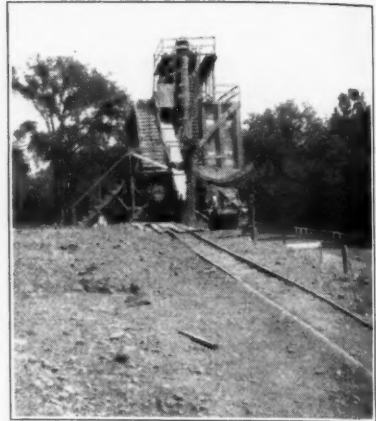
The Crushing and Screening Plant Showing the Railroad Approach to the Plant.
